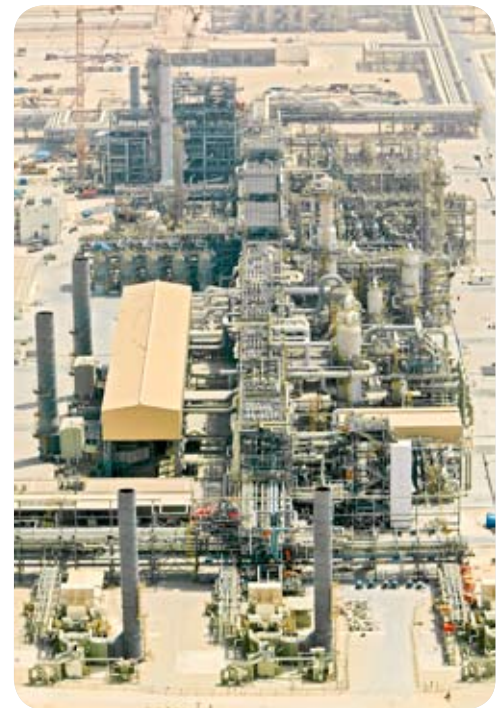
Train 3, the first train under the RasGas Expansion Project
